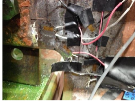
(b) Stringer cope of the lab specimen
