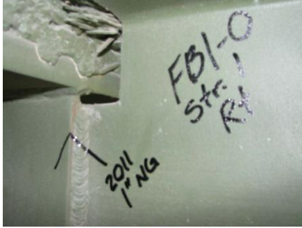
(a) Stringer cope of an existing bridge
