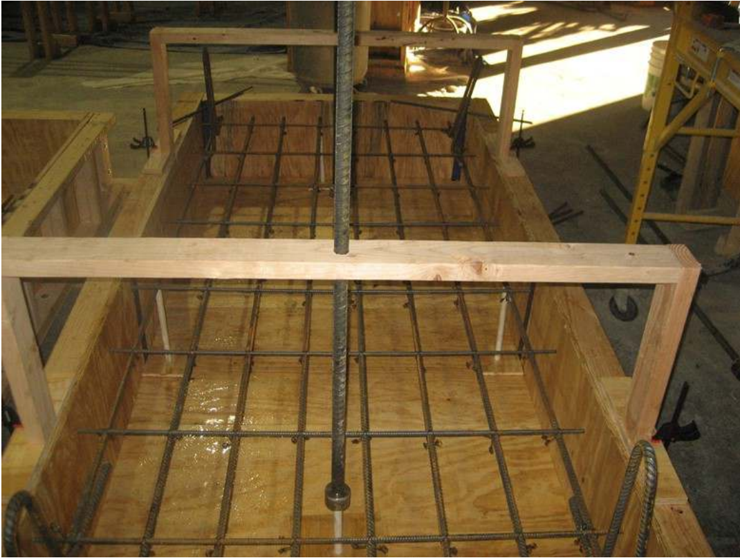
Figure 3.6 Slab specimens in Series 1 and 2 that contained No. 4 and No. 5 bars perpendicular to the headed bar distributed evenly along the long and short direction of the specimen
