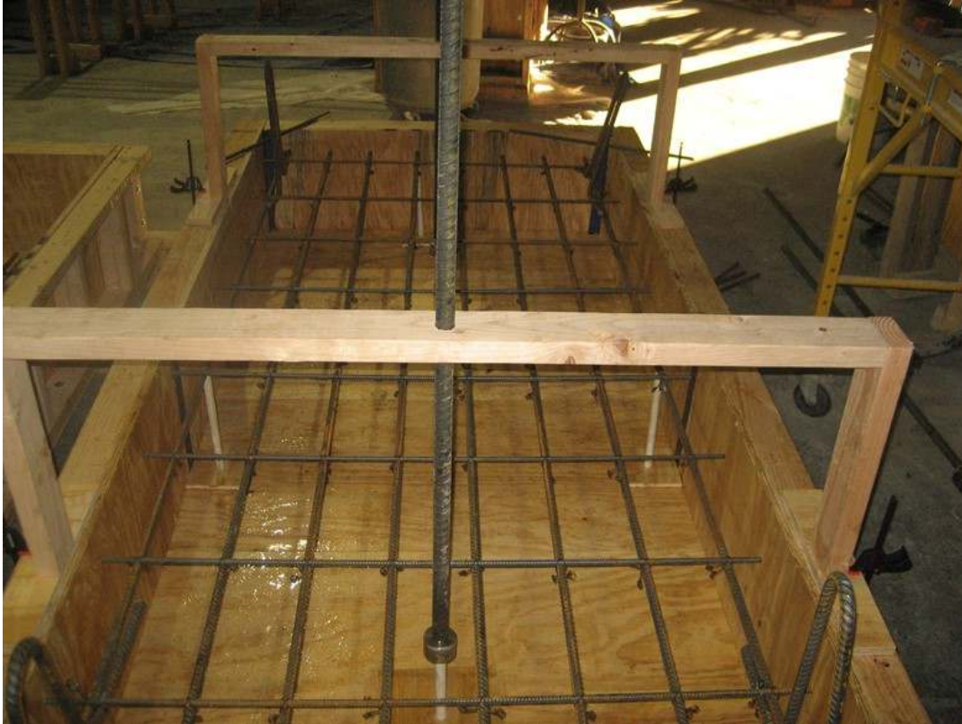
Figure 2.6 Slab specimen formwork
