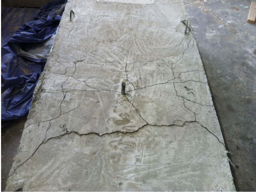
Figure 3.1b Breakout failure of slab specimen 8-5-F4.1-6#5-6 from test Series 5 with both supports outside the failure region (specimen contained a single bar anchored at the middle of the slab)
