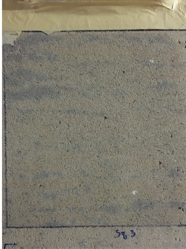
Figure 2.7: Concrete surface prepared to Concrete Surface Profile 3 (CSP-3)
