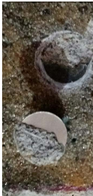
Figure 2.12: Pull-off test exhibiting 60% concrete substrate failure and 40% glue failure
