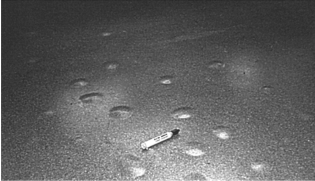
Figure 1.1: Blistering under a floor covering (ACI 302.2R-06)
