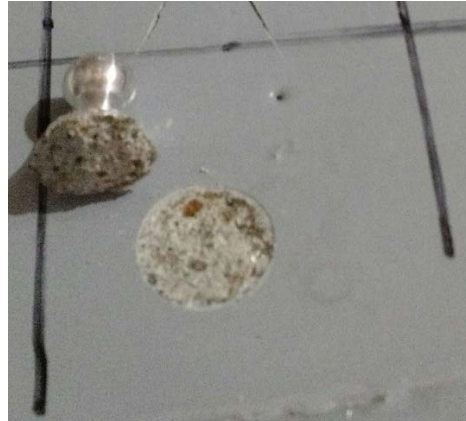
Figure 2.9: Pull-off test exhibiting concrete (substrate) failure
