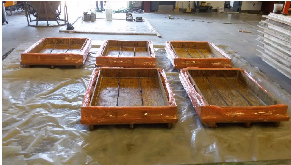
Figure 2.4: Slab specimen formwork
