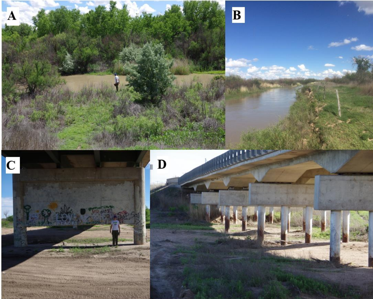
Figure 19: Examples of evidence for channel entrenchment at four locations within the study area reach: A) author standing on the former braided channel bed, B) the change in elevation of the river flowing east near Kendall, C) author standing on the present-day channel bed (dry); when the Garden City West Bridge pilings were emplaced in 1957 the channel bed was at the base of the cross panel between the support columns (entrenchment of about 1.5 m), and D) Pierceville Bridge with similar conditions to that of C.
