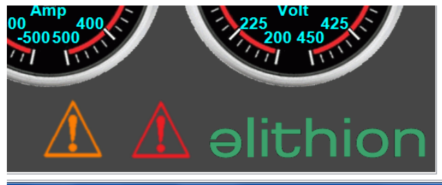
Figure 129: While viewing the meters tab, a fault is indicated by a red exclamation mark. The orange exclamation mark indicates a warning is present.
