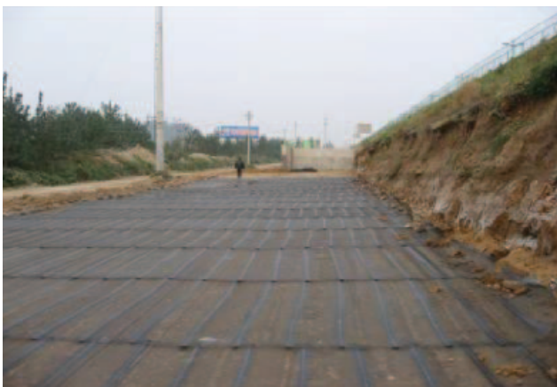
Figure 17. Photograph showing an installed geogrid under the widening embankment
