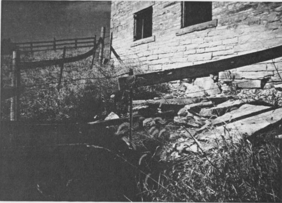
Figure 3.35 Runoff pipe from spring room to stream feeding Mill Creek
