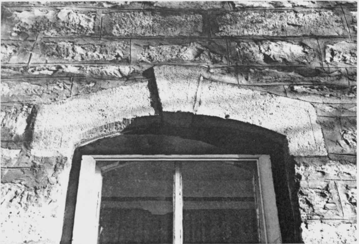
Figure 3.24 Detail of stone lintel with keystone
