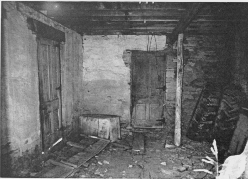
Figure 3.36 View through east door of kitchen, Grimm spring house
