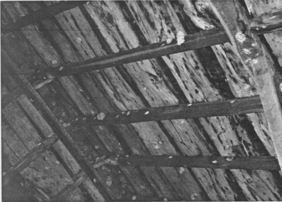
Figure 3.17 Double roof structure, Henry Grimm barn
