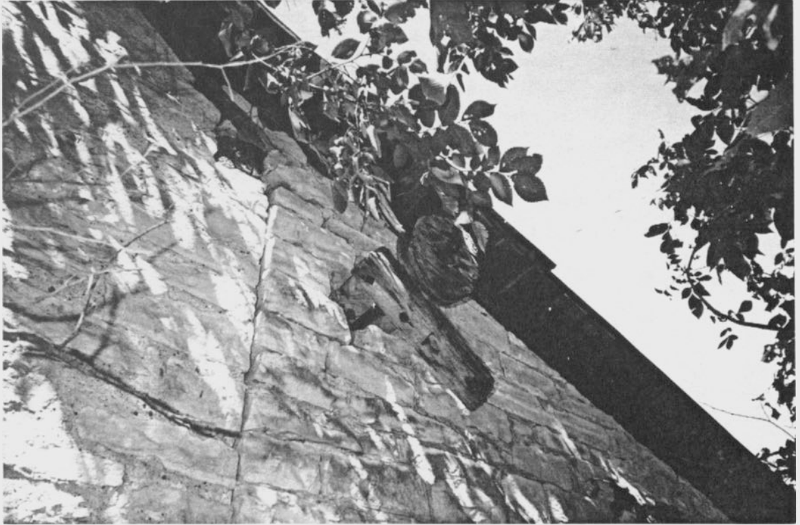
Figure 3.42 Exterior view, hoisting mechanism to Grimm wash house
