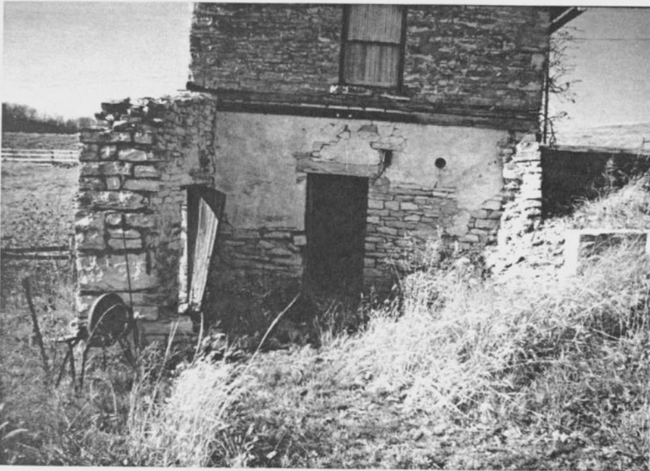
Figure 4.22 Remains of previous open-air covered kitchen off of the east end of the spring house
