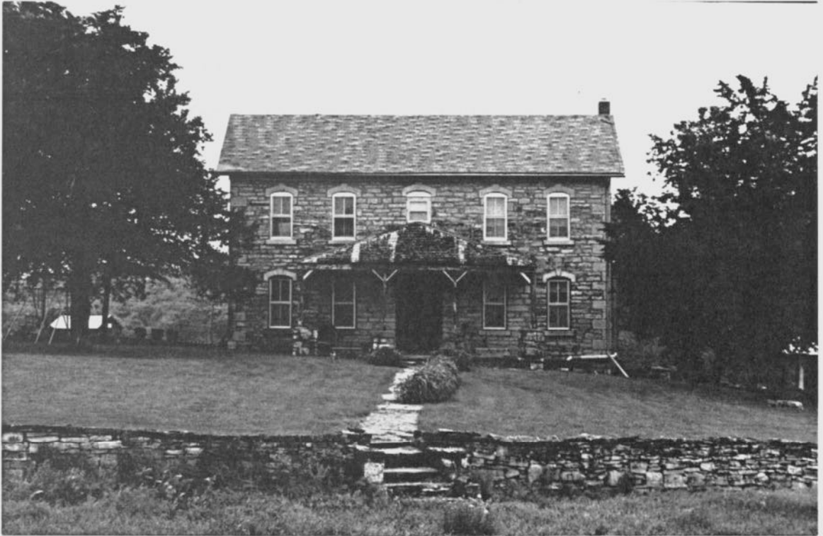
Figure 6.7 Bill and Mary Schultz's one-story porch addition to I-house
