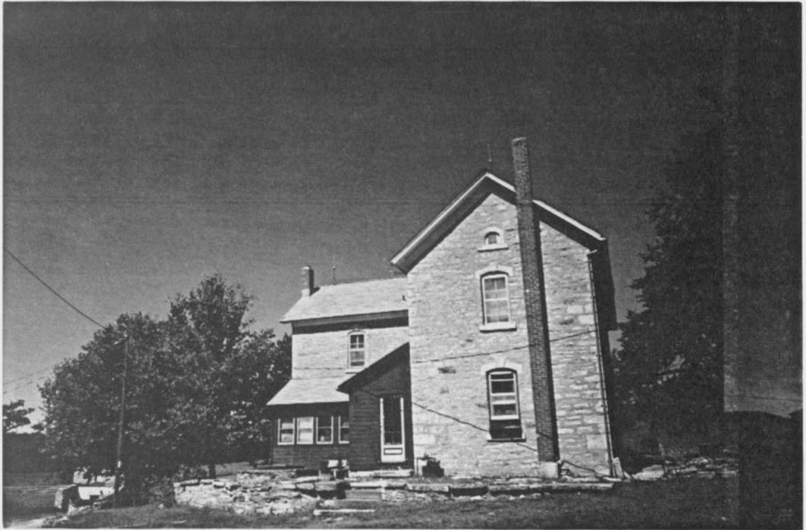
Figure 4.21 View of porch ell addition from east, Henry Grimm I-house
