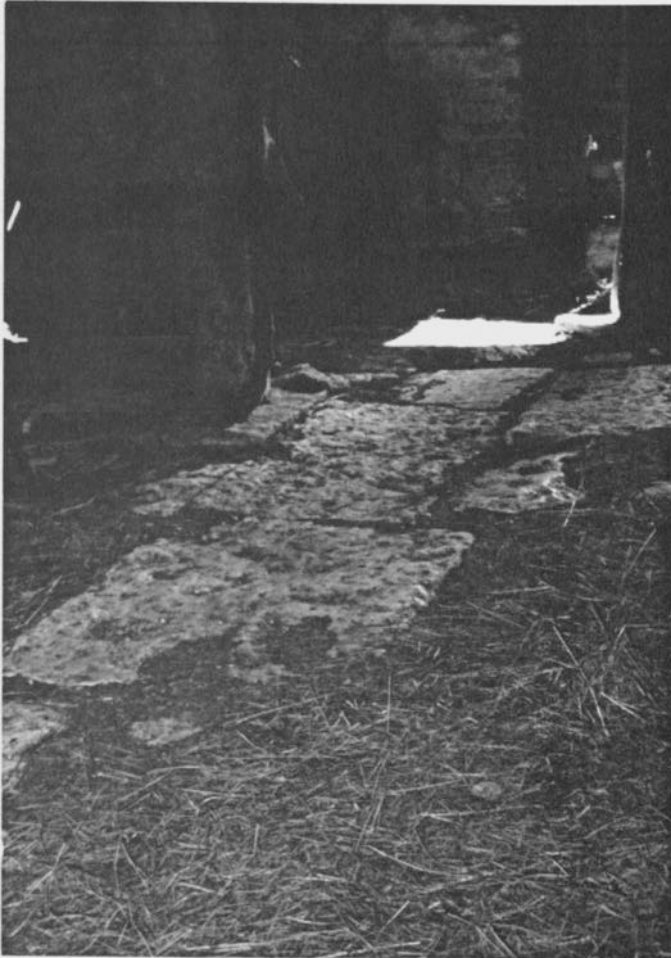
Figure 3.12 Limestone paving and view of tack room, central Grimm barn
