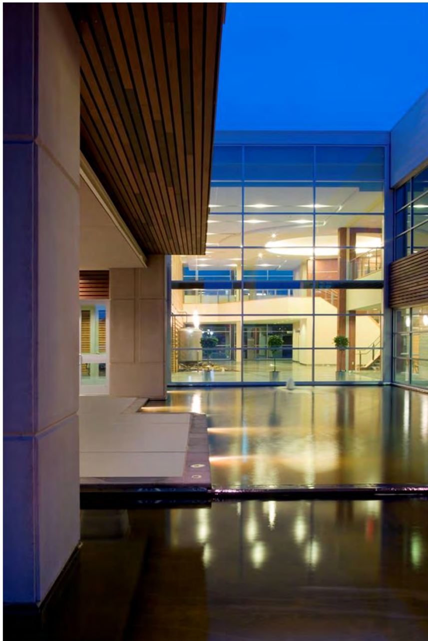
Figure 3: The reflecting pool at the entrance of the building works as a retention pond.
