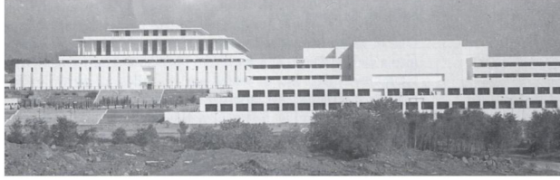
Figure 10 Stone's Parliament Building (right) and President's Secretariat (left) (Source: Architecture in Pakistan)
