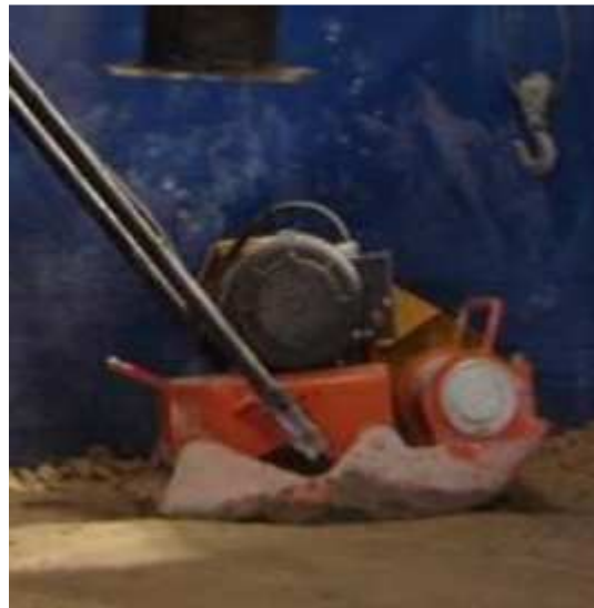
Fig. 4.3.3 Compacting subgrade using the vibratory plate compactor
