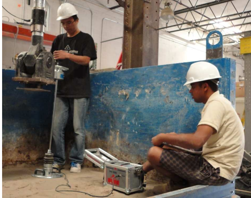
Fig. 5.3.3 Light Weight Deflectometer (LWD) test on subgrade
