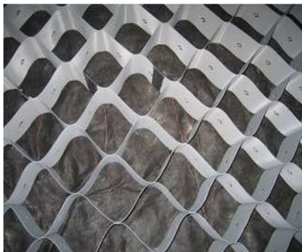
Fig. 4.3.8 Installing geotextile and geocell on top of subgrade
