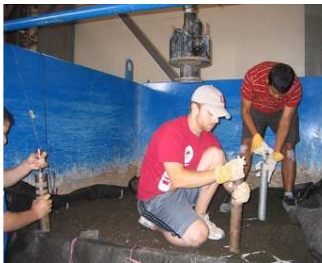
Fig. 4.3.9 Compacting RAP inside geocell pocket using hand tamping
