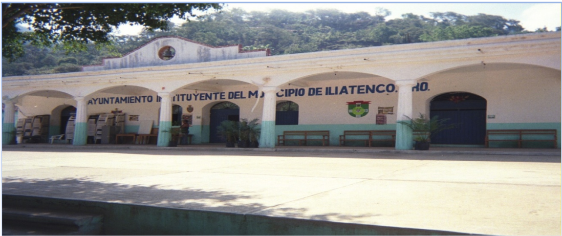
Figure 4 The ayuntamiento (town hall) in the central plaza of Iliatenco is the municipal administrative center. Before 2005, this building was a comisaría to the ayuntamiento in Malinaltepec. (Photo by David López)
