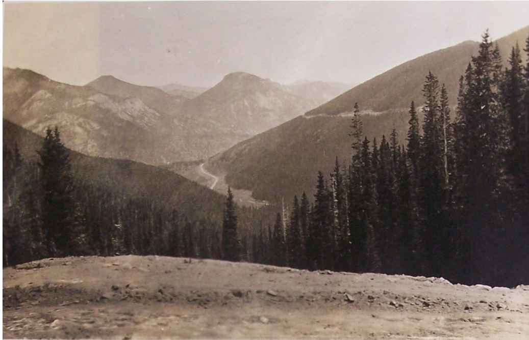
View of newly constructed Trail Ridge Road and surrounding mountains. (Photo by Charles V. Dunn, 1932)
