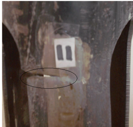
Fig. B9 - Monotonic Tension, Fracture Failure Close View from Outside.
