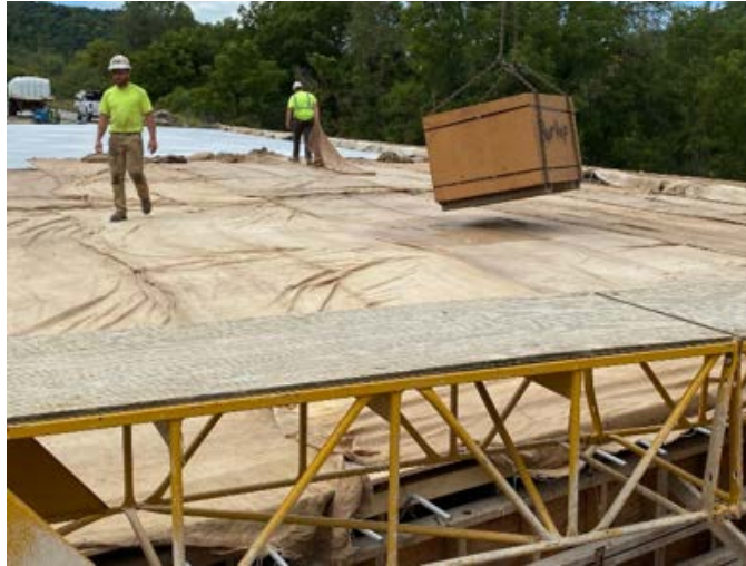
Figure 2.40: Wet Curing Application on MN-IC-LC-HPC-9
