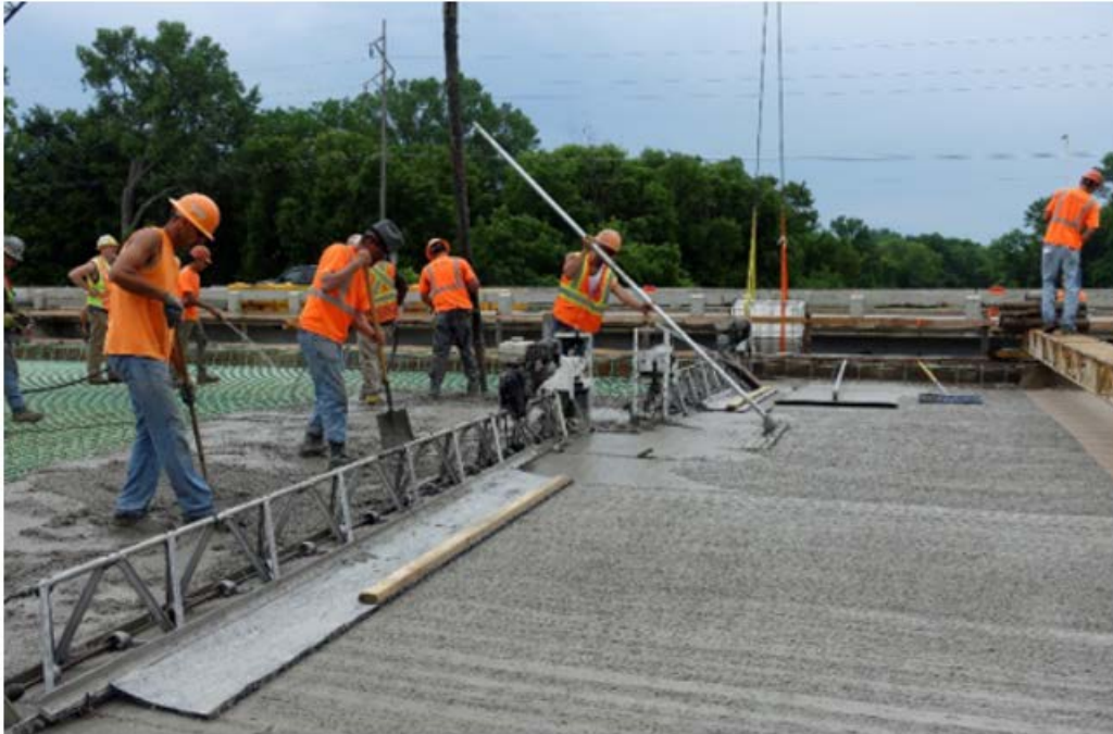
Figure 2.3: Finishing Equipment for MN-IC-LC-HPC-2 Subdeck
