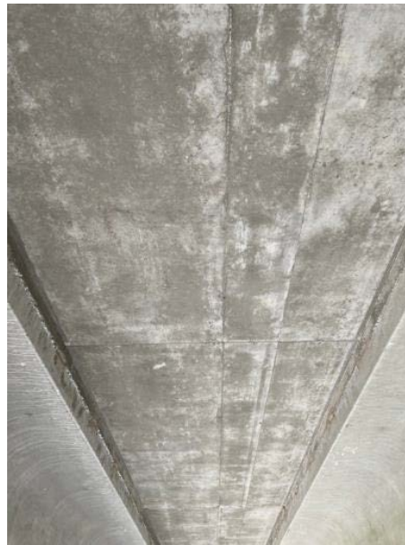
Figure 3.29: Underside of MN-IC-LC-HPC-9 Bridge Deck
