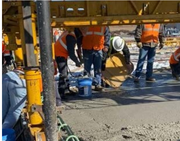
Figure 2.58: Applying Finishing Aid to the Concrete Surface
