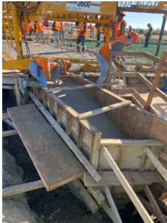
Figure 2.51: Walking Observed on Freshly Consolidated Concrete
