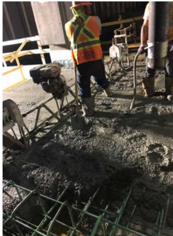
Figure 2.10: Placement, Consolidation, and Finishing of MN-IC-LC-HPC-5
