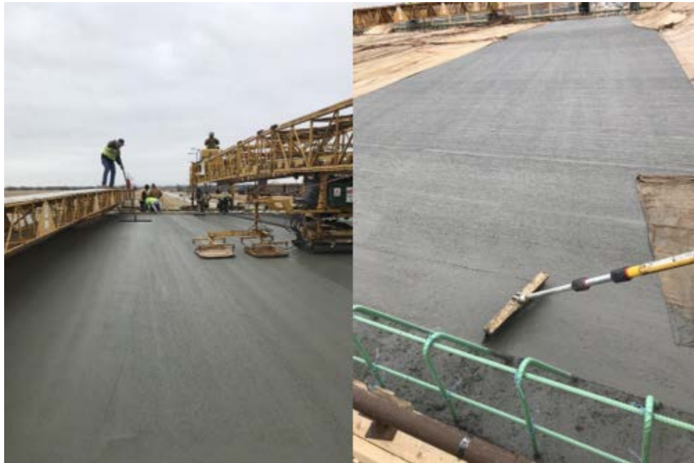
Figure 2.47: Bull Floating and Brooming (a) Bull Floating the Deck; (b) Brooming
