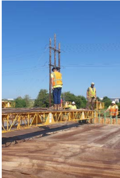
Figure 2.68: Rewetting the Burlap on the Deck
