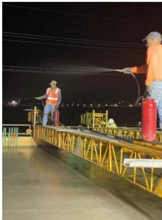
Figure 2.66: Applying Finishing Aid to the Concrete Surface
