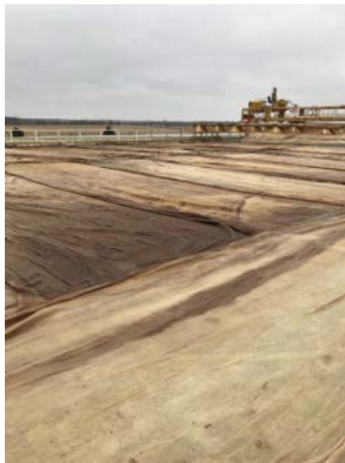
Figure 2.48: Burlap Placement on the Deck
