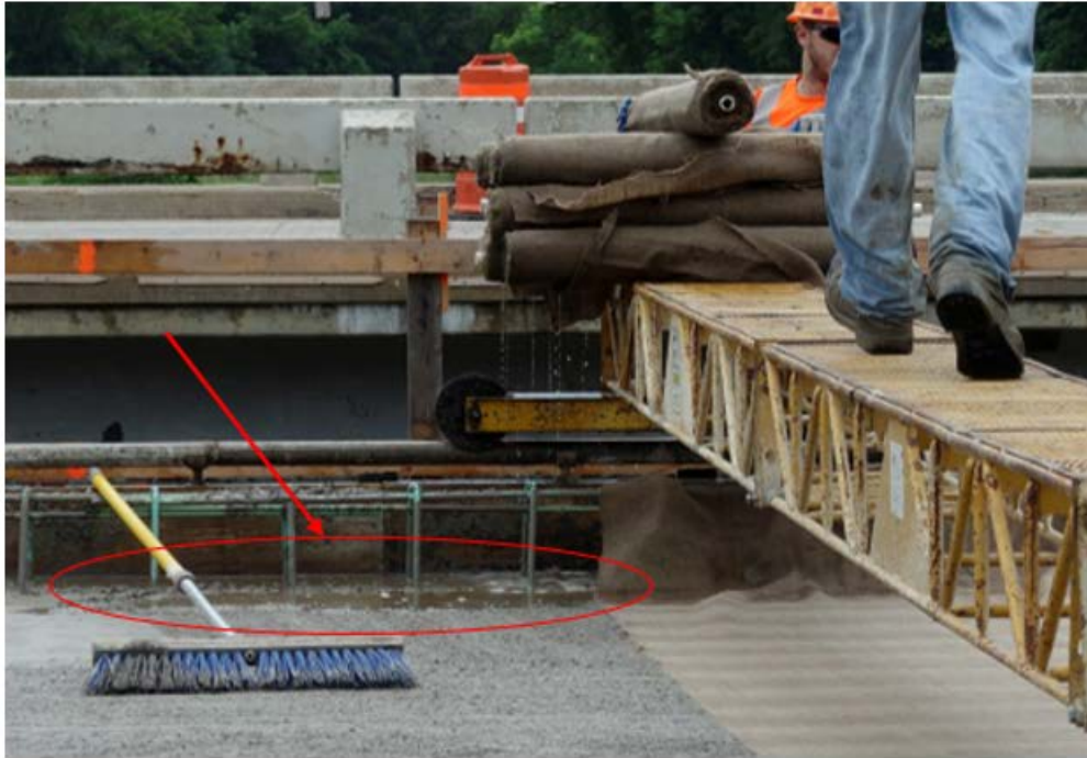
Figure 2.4: Water from Burlap Dripping onto the Deck
