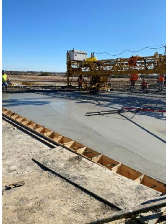
Figure 2.53: Over-Finishing the Deck in the Presence of Bleed Water
