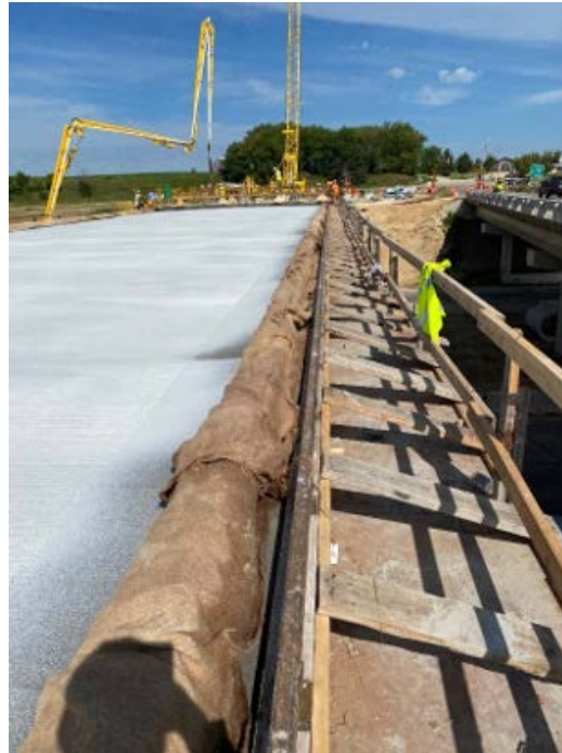
Figure 2.33: Burlap Placement on the Barrier Reinforcement
