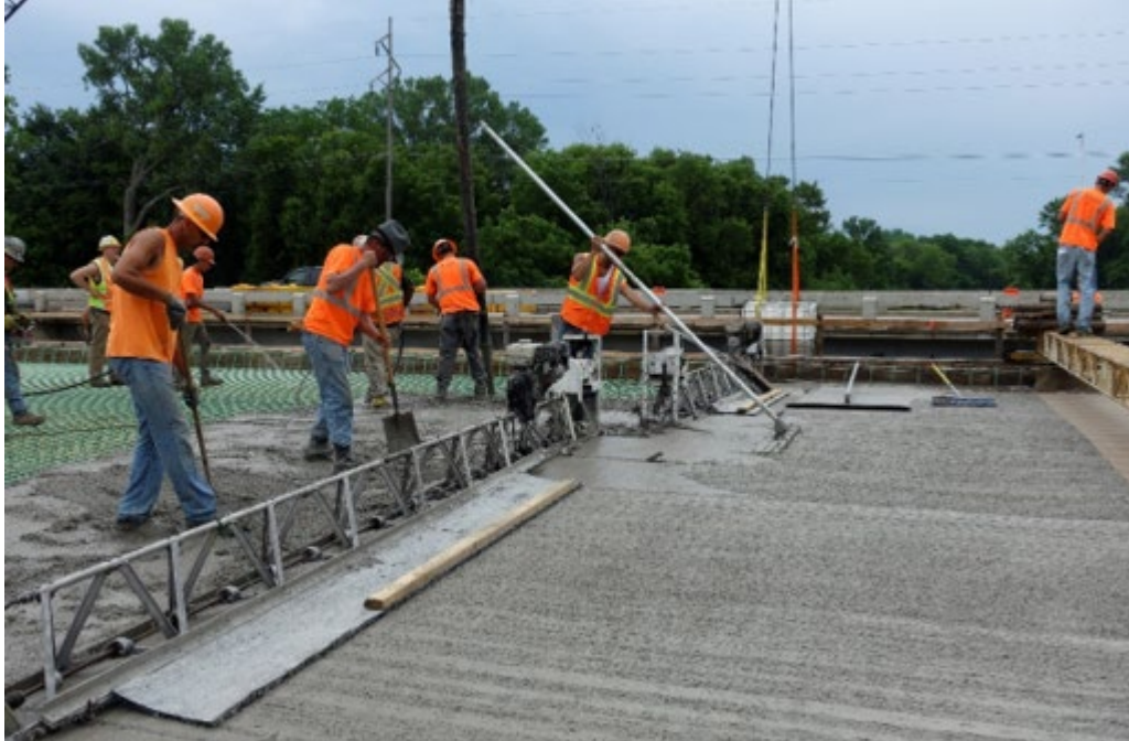
Figure 4.2: Finishing equipment for MN-IC-LC-HPC-2 subdeck
