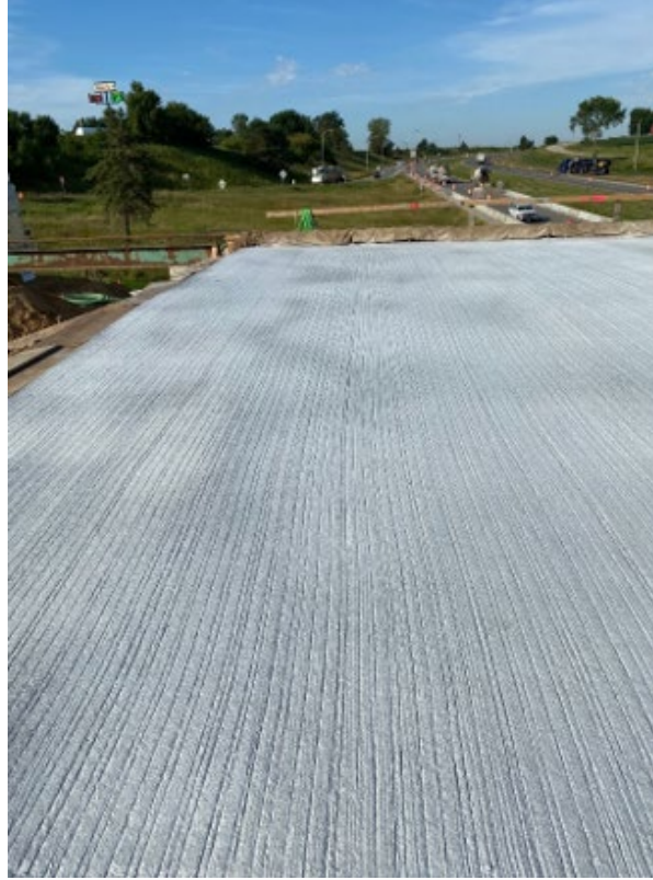
Figure 4.31: Non-uniform distribution of curing compound on the deck
