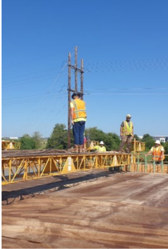
Figure 4.68: Rewetting the burlap on the deck
