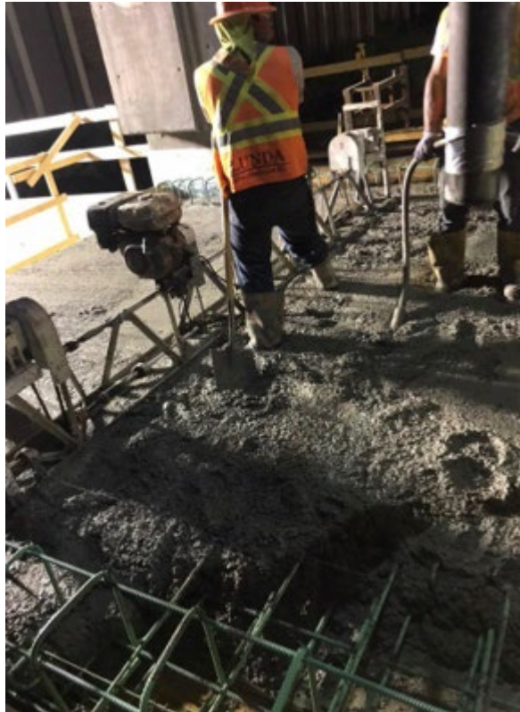
Figure 4.9: Placement, consolidation, and finishing of MN-IC-LC-HPC-5
