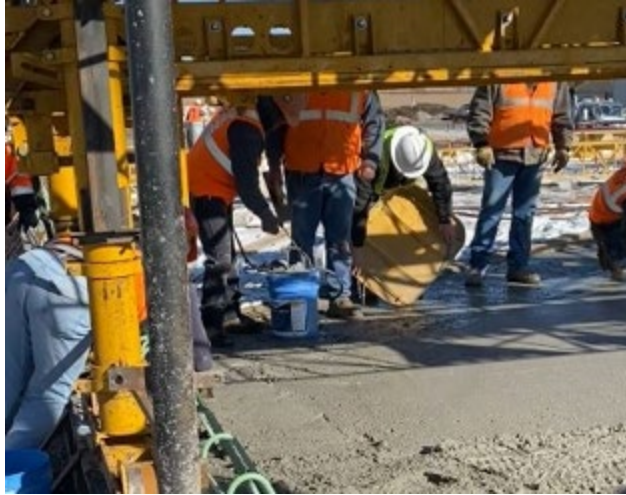
Figure 4.58: Applying finishing aid to the concrete surface
