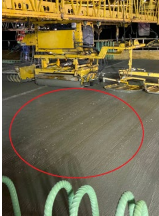
Figure 4.65: A leaking pipe leaving water droplets on the deck surface
