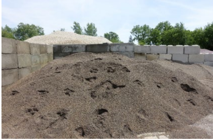
Figure 4.1: Lightweight aggregate stockpile for MN-IC-LC-HPC-2
