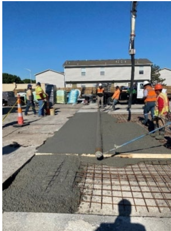
Figure 4.63: The qualification slab placement equipment
