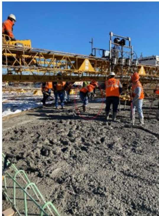
Figure 4.56: Walking observed on freshly consolidated concrete
