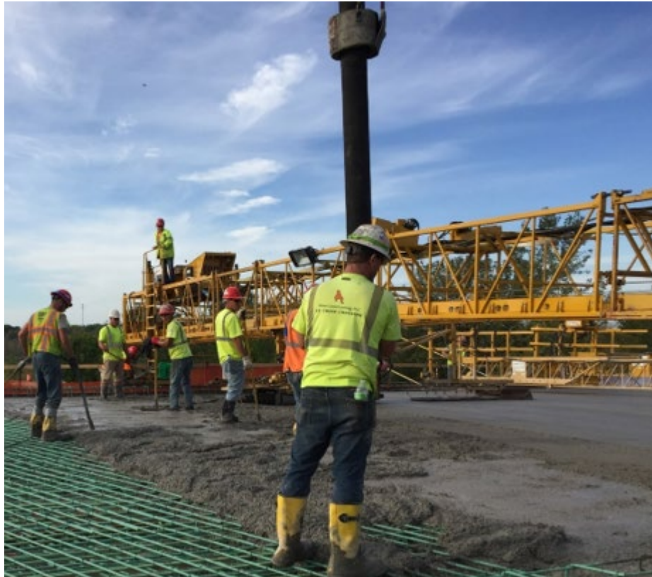
Figure 4.16: Placing, consolidation, and finishing equipment
