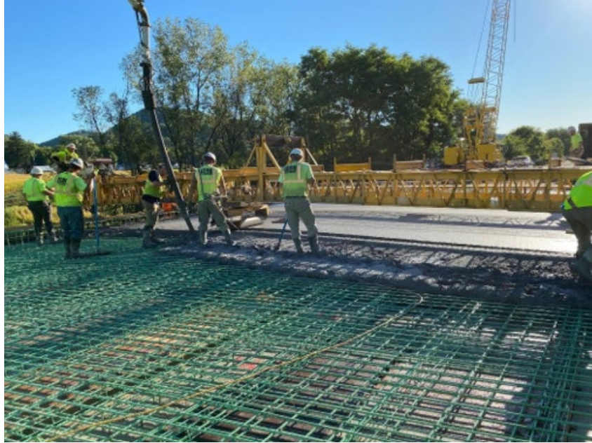
Figure 4.35: MN-IC-LC-HPC-9 placement
