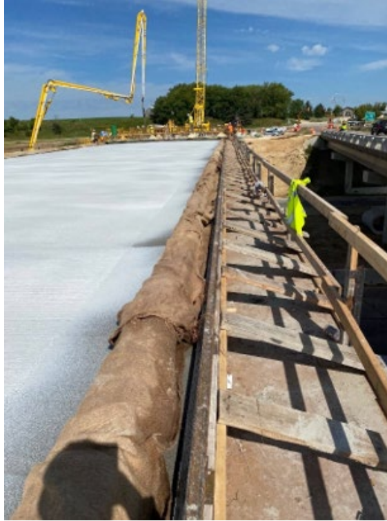
Figure 4.32: Burlap placement on the barrier reinforcement
