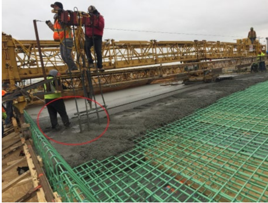
Figure 4.46: Walking through consolidated concrete
