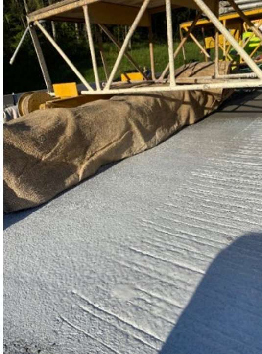
Figure 4.37: Burlap placement on the barrier reinforcement
