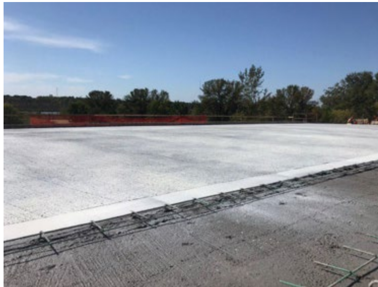
Figure 4.19: The application of the curing compound on the roadway of the deck
