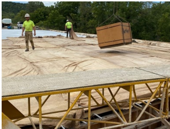
Figure 4.39: Wet curing application on MN-IC-LC-HPC-9
