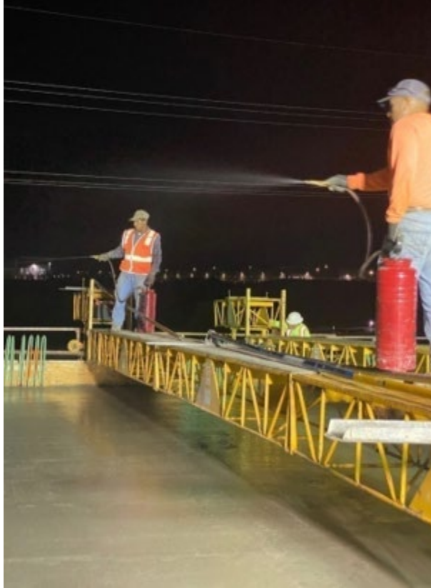
Figure 4.66: Applying finishing aid to the concrete surface
