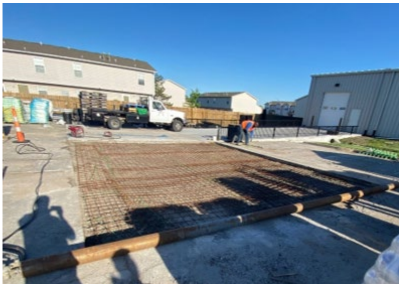
Figure 4.62: The qualification slab for KS-IC-LC-HPC-3
