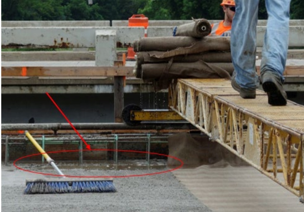
Figure 4.3: Water from burlap dripping onto the deck
