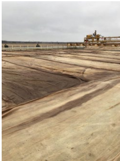
Figure 4.48: Burlap placement on the deck
