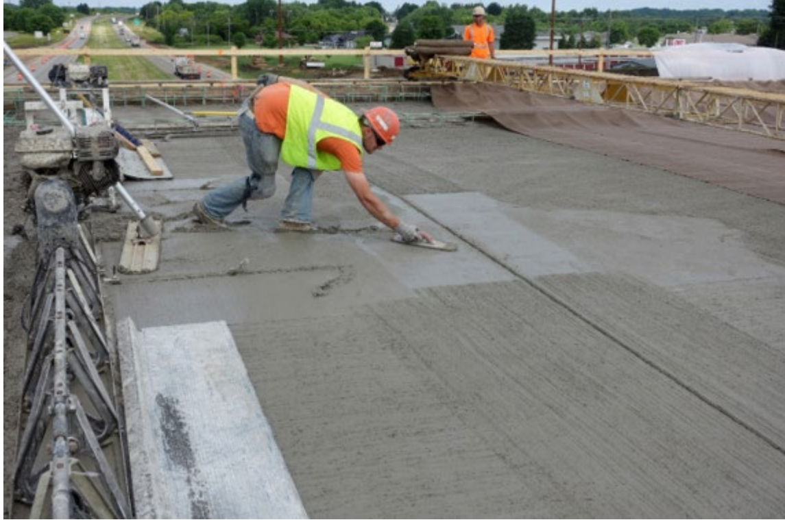
Figure 4.4: Walking through freshly consolidated concrete
