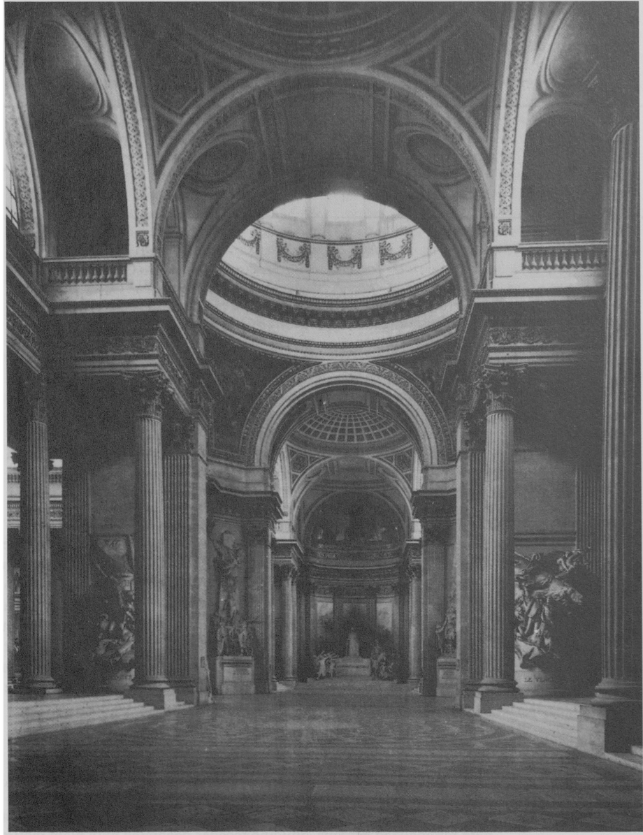
FIGURE 2-1 Soufflot, Ste-Geneviève (now the Panthéon), Paris, 1755–90; crossing piers strengthened by Rondelet in 1806. [Photo used by permission of A. F. Kersting]
