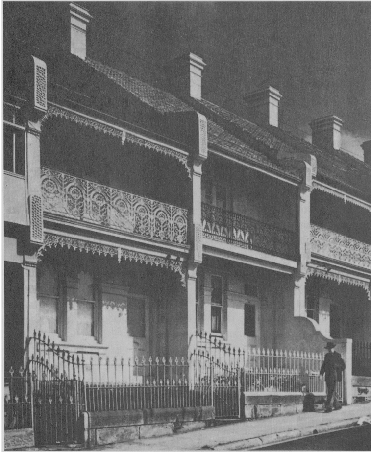
FIGURE 10–6 Terrace housing, Sydney, Australia; structural sun-shading of street fronts. [Photo used by permission of Max Dupain and Assoc.]
