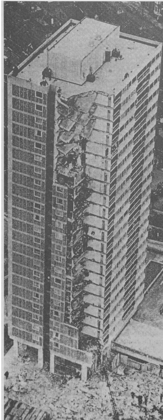
FIGURE 6-8 Roman Point, London. [Used by permission of Built Environment ]
