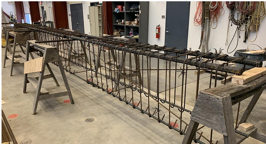
Figure 3.4: Reinforcement after assembly (18-a)
