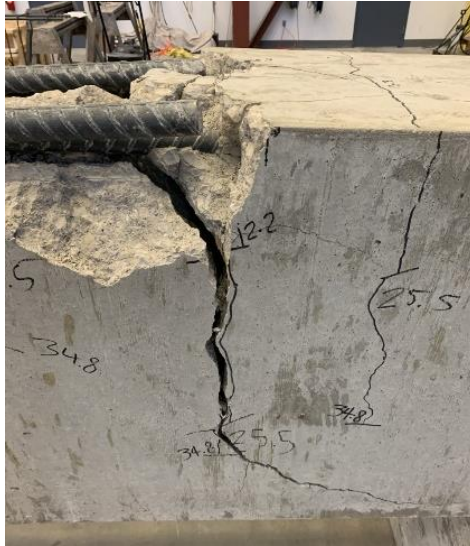
Figure 4.6: Unconfined lap splice failure (14-a)
