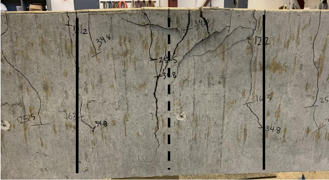
Figure E.3: Photo of 14-c after failure
