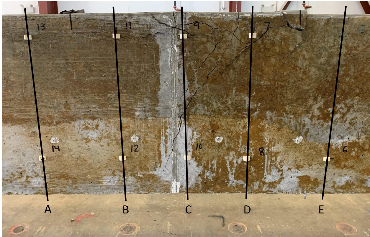
Figure G.5: Specimen 18-d with inclined crack spanning from the compression fibers in B-C to the D-E tension face after failure
