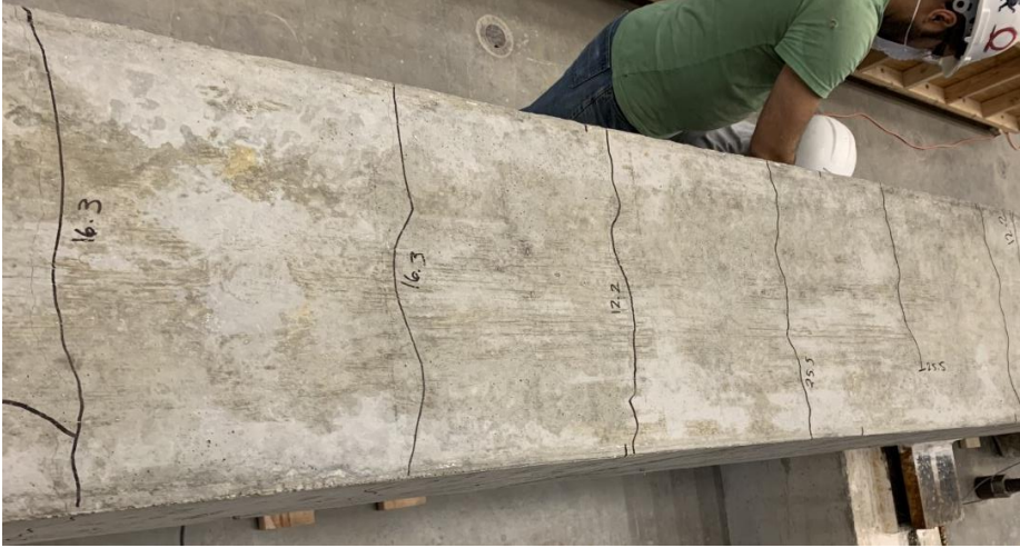
Figure 4.2: Cracking along transverse reinforcement on tension face (14-b)
