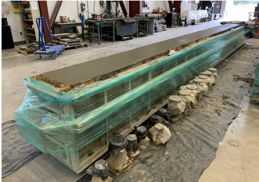
Figure 3.7: Formwork after concrete placement (14-b)
