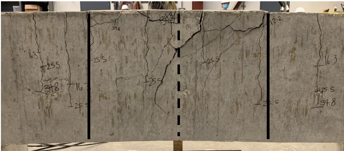
Figure E.2: Photo of 14-b after failure
