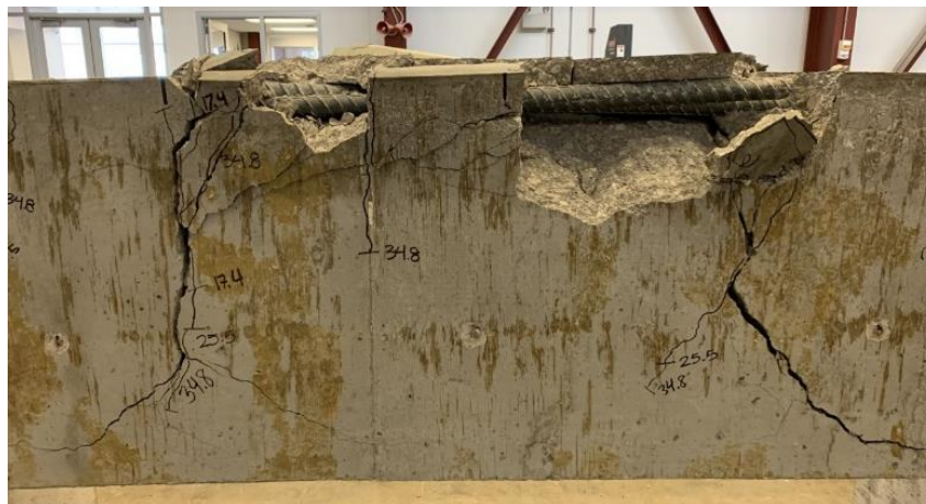
(c) After failure
