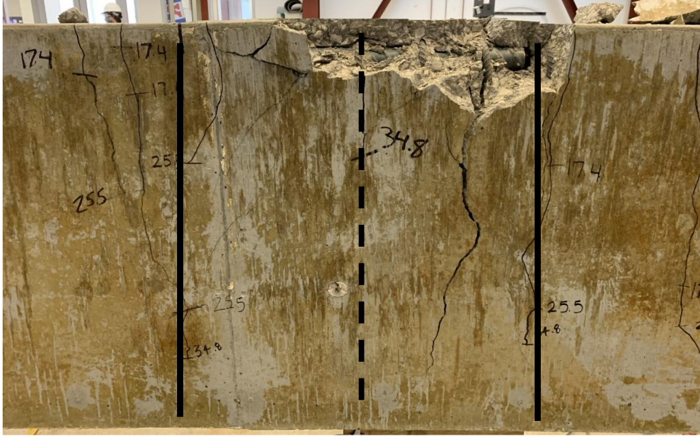
Figure E.5: Photo of 14-e after failure
