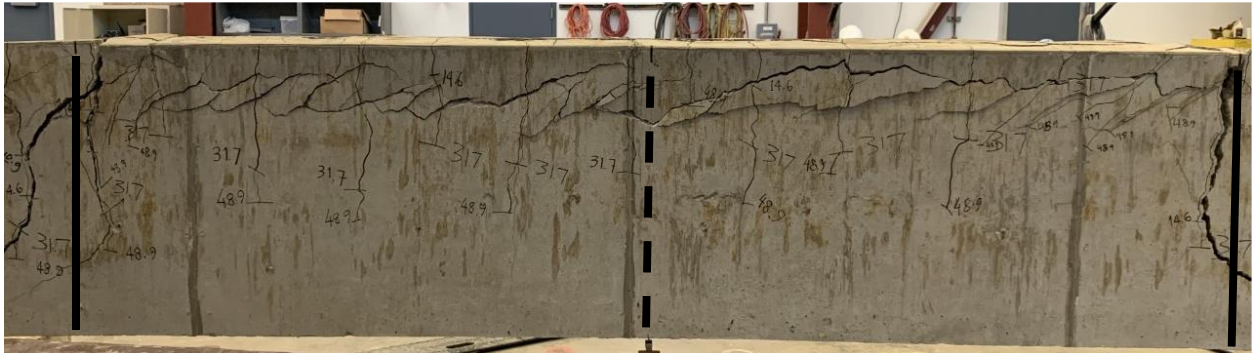
Figure E.6: Photo of 14-f after failure
