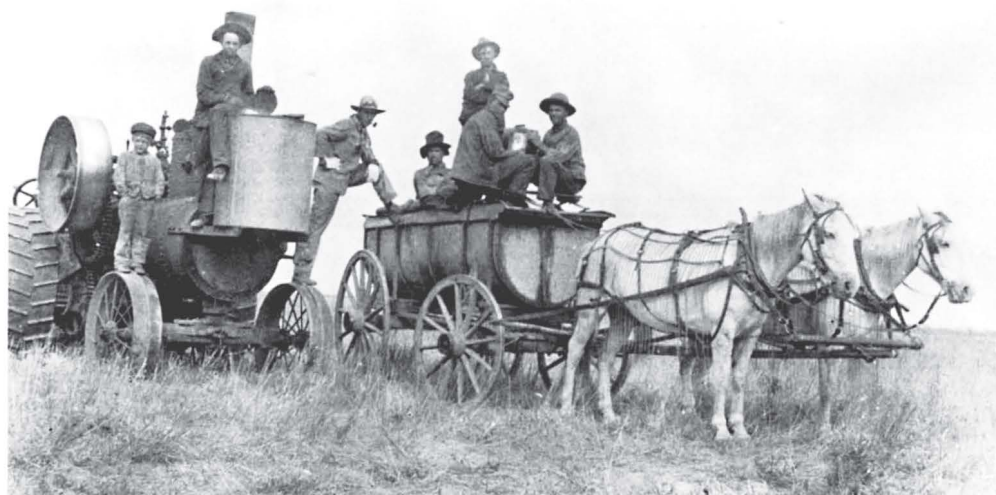
Hauling water back to fill the reservoir (here with an extra front-mounted tank, optional on Minneapolis engines) on the engine, the tank man might also bring some for the hands, such as these on the R. Doris crew, Lane County, Kans. (Lane County Historical Museum, Dighton, Kans.)
