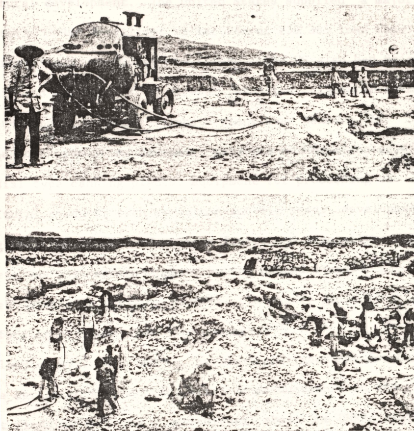
Fig. 6. Rock for the dike across the main channel was obtained from a quarry 60 miles from the job. American air compressors and rock drills were used, being in charge of an experienced American operator.
