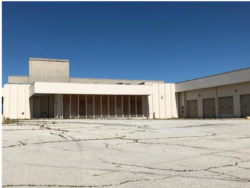
Figure 1.2 Former Sears Building in Leavenworth, Kansas
