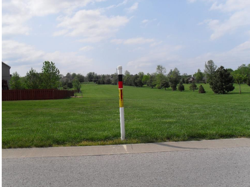
Figure 2.18: Pipeline running through Leavenworth County, Kansas
