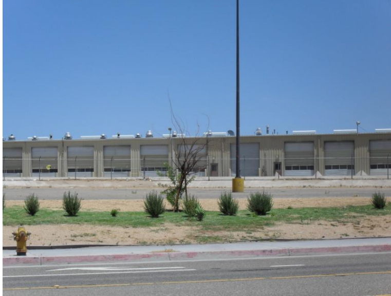
Figure 7.1: Cross Docking and Trans-loading Facility—Located near Major East-West and North-South Roads and Major Rail Yard
