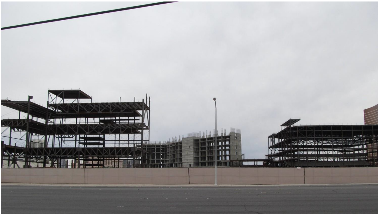
Figure 8-1a: Major Construction Project in Las Vegas Started in 2008 - Projected Completion 2021
