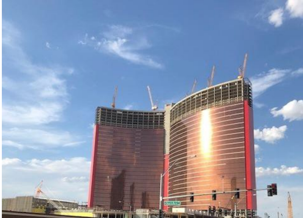
Figure 8-1b: Status of Building as of February 2020
