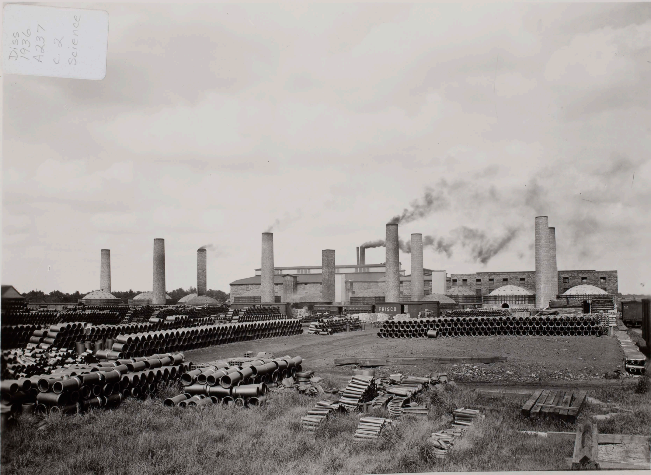
Fig. 13.--Pittsburg plant of the W. S. Dicky Clay Manufacturing Company.
