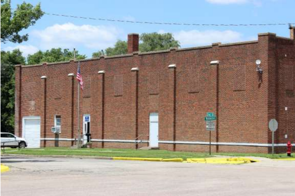
Photo 6: Side View of the Old City Office/Auditorium
