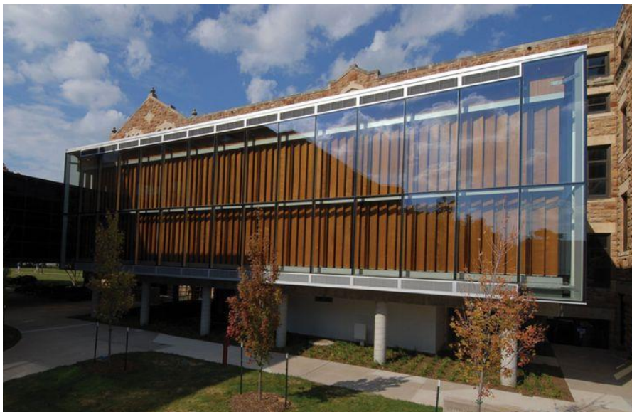
Figure 3.1 The Forum at Marvin Hall designed and constructed by Studio 804
