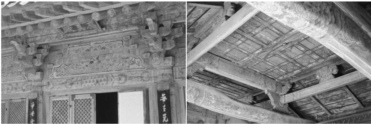
The bracket complex of the Eungjin-jeon: the Jusimpo type
