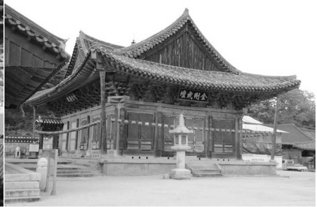
View of the southwestern side of three-gabled roof
