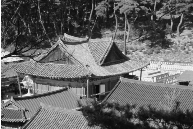
View of the southeastern side of three-gabled roof
