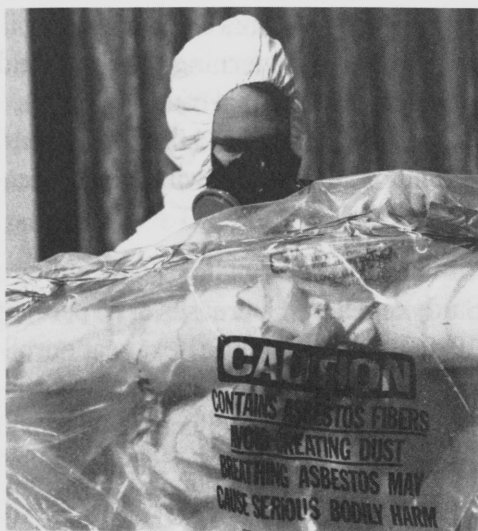
A student in protective garb learns 'glove-bag' asbestos removal techniques during an NATC-sponsored training session in 1987.
