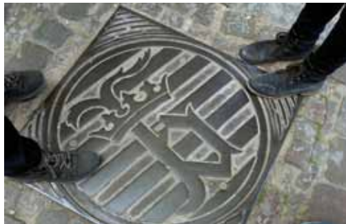
Figure 10: A sewer pipe cover in Bruges, Belgium.
