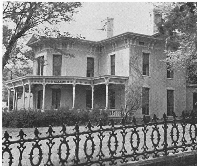
TEMPLIN HALL, the first men's scholarship hall, was the result of a campaign led by Dean Olin Templin. Now vacant, it's due for bulldozing to provide space for new apartments for retired faculty.
