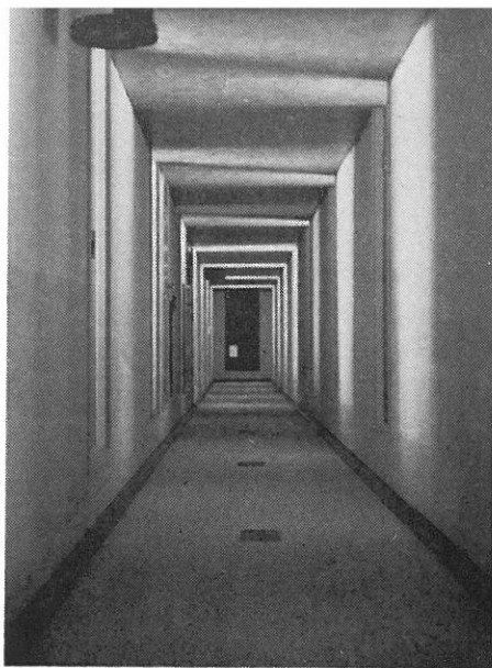
CONNECTING HALLWAYS join the individual rooms in each 36-man unit of J.R.P.
