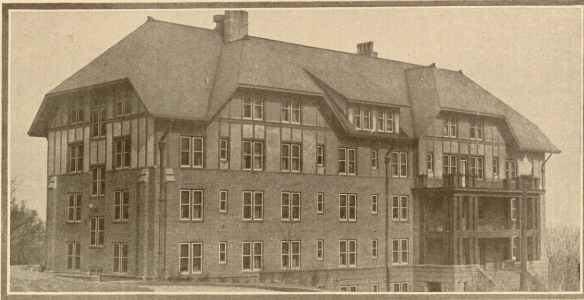
Corbin Hall Was First State Dormitory for Women
