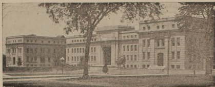
ADMINISTRATION BUILDING, UNIVERSITY OF KANSAS
